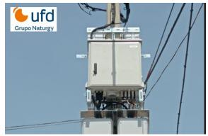
phases by means of distributed equipment installed in an LV network. This system provides a scalable solution by adding as many LV Network Smart Balancers as required and foresees continuous communication to analyse data, algorithm adaptation, diagnosis, and integration of other functionalities (such as energy storage management) in remote and advanced network monitoring.
