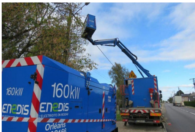
Live work reducing the impact of work on customers.
